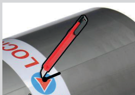
Cutting halfway through the adhesive strip
